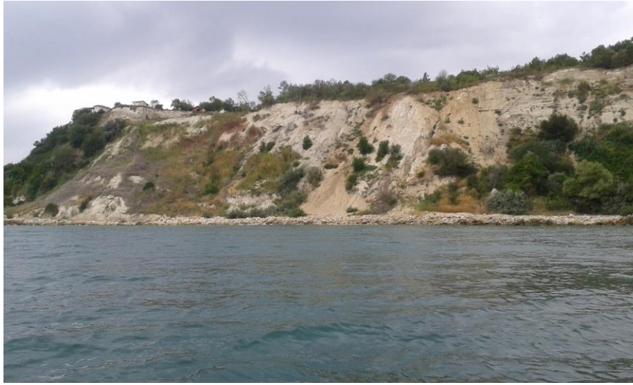
Figure 1. General view of landslide toe.
