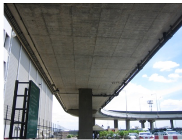
(a) Viaduct at Don Muang Airport (1998)
