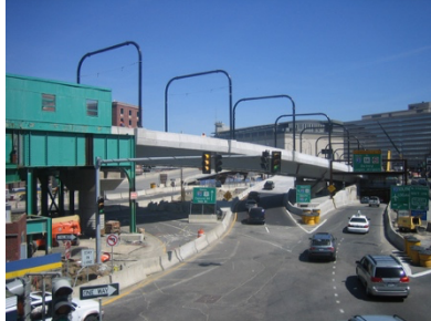
(a) MBTA Green Line viaduct, Boston
