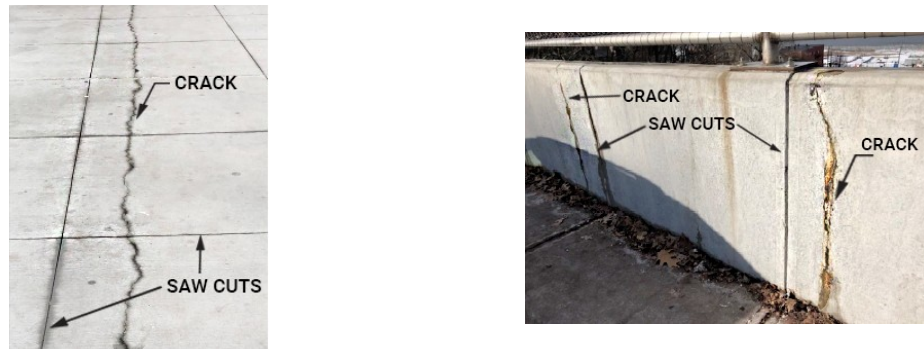
(a) Concrete sidewalk on Park Ave., NYC
