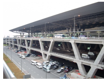
(b) Viaduct at Suvarnaphoom Airport (2005)
