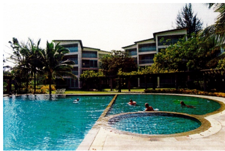
(a) Chom-View Condominium
