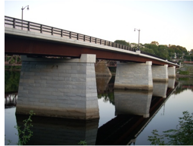
(b) North Adams Bridge in Haverhill
