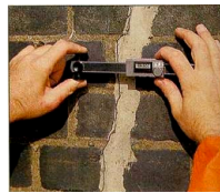
Figure 5. Using a Crack Measuring Gauge (Avşar et al. 2014).
