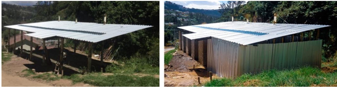
Figure 1. The initial independent structure is on the left, and the eco earth sandwich enclosure is on the right.
