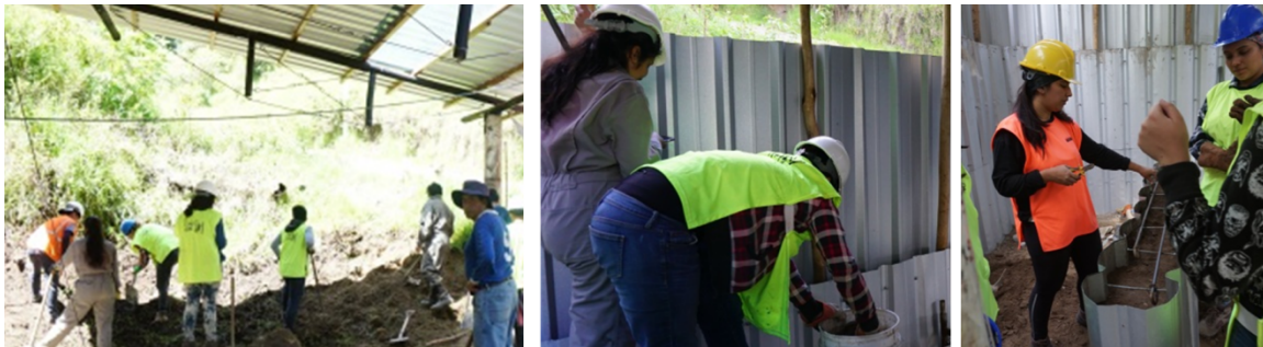
Figure 1. Community and students during the construction process.
